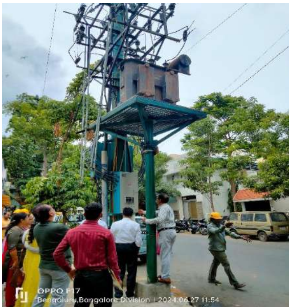
Overhead Distribution Transformer
