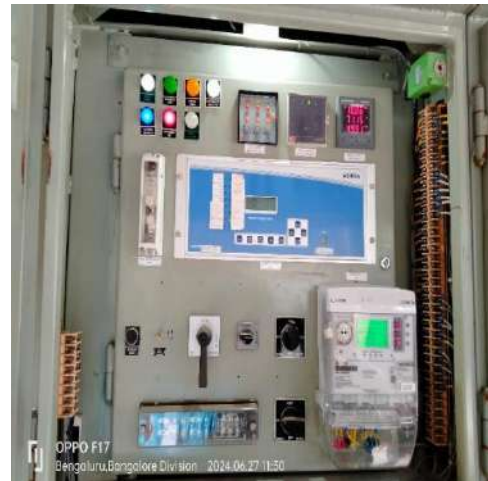
Energy Meter, Control & Annunciator Panel (Feeder 1)
